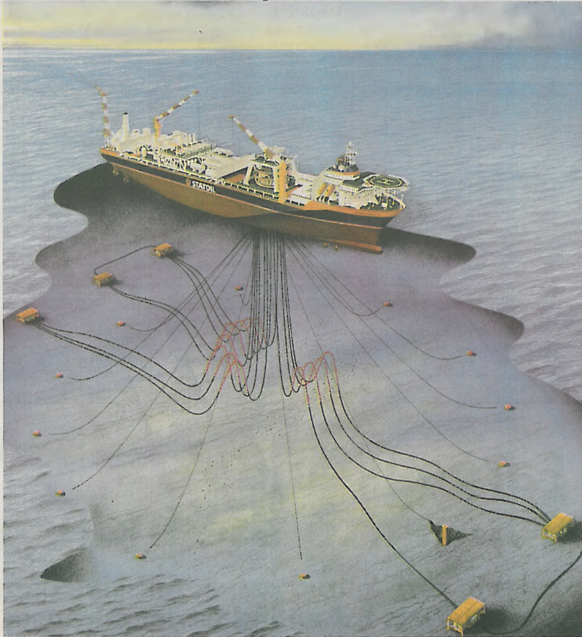
Production and cargo ship in the Norne Area in Northern Norway with sub-sea units producing 200.000 barrels a day
